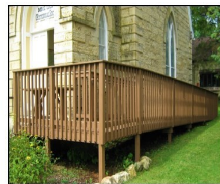
The ramp at the historical society was repaired and restained.
