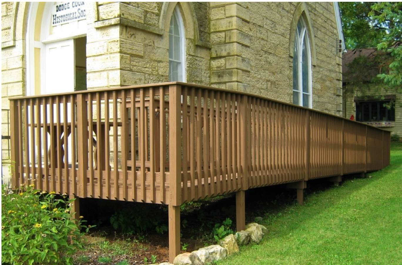
The access ramp (above) and robing room stairs (below) at the museum got a new lease on life after sanding and staining.
